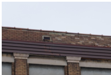
Metal flashing on parapet.
